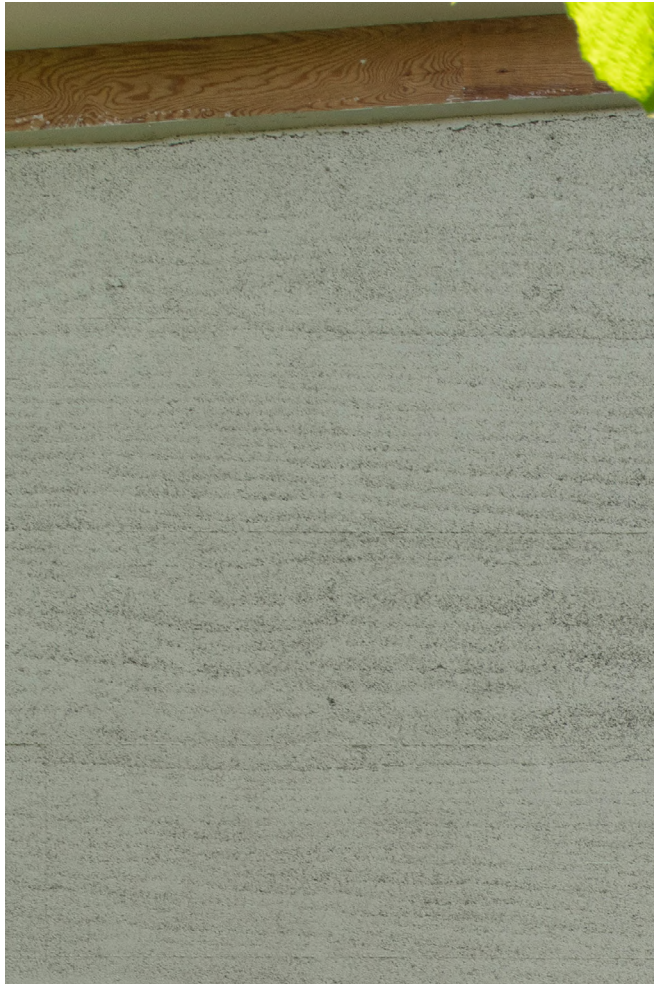
The rammed hempcrete visible texture
