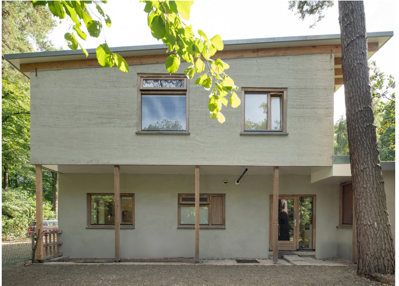
The western façade features hempcrete for both insulation and finish, paired with a timber structure
